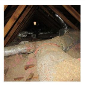
The duct supplying the family room (garage) is disconnected. We review and repairs.
