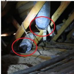
Duct/boot for front bedroom is loosely installed and leaking into the attic space; we recommend review and repairs as needed.
